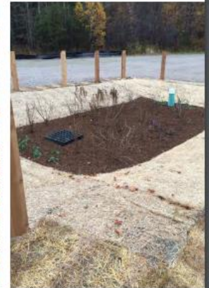
Before, left, and after, right, the installation of a bioretention stormwater treatment structure at the Lake Iroquois public beach parking lot. The project was completed by the Lake Iroquois Recreation District with support from an Ecosystem Restoration Grant.
